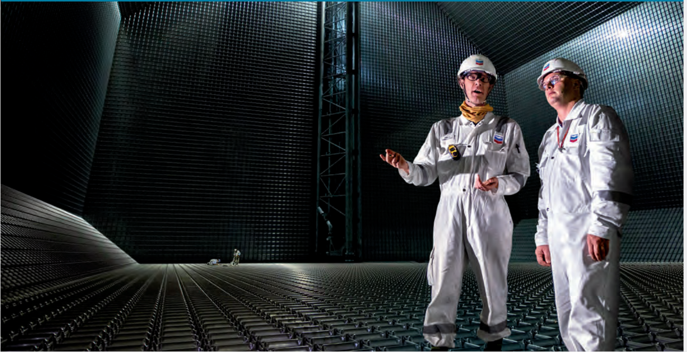
Chevron Shipping Company employees inspect a liquefied natural gas (LNG) storage tank under construction in South Korea during the company's largest shipbuilding and fleet modernization program in corporate history. The program included delivery of seven new ships to support growing LNG operations.
